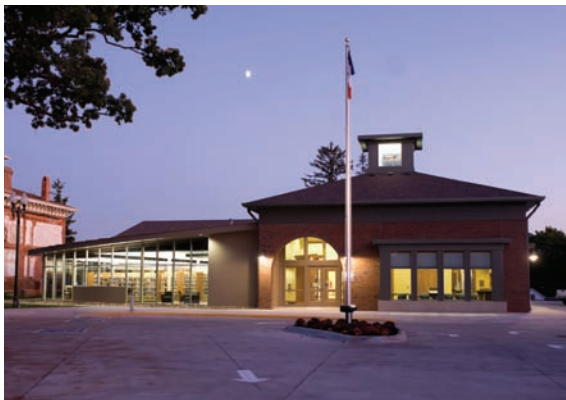
ECI REC assisted Independence in building its new library, completed in September 2008.
